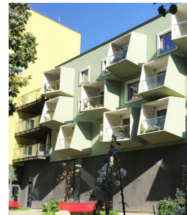
Clustered units with balance between private and communal living. Health services on ground floor, Ørestad, Copenhagen.
